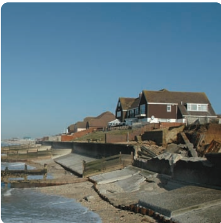
Left: Damaged sea defenses, Selsey, United Kingdom
