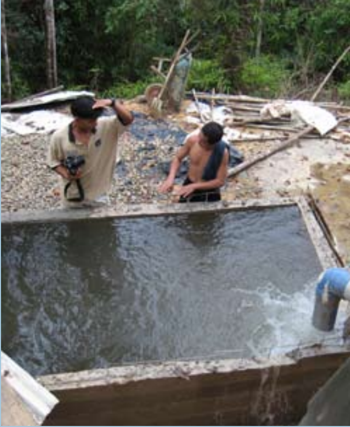
Community members of Terian, Sabah, Malaysia repair the water catchment above their microhydro generator. Image: Shawn Sullivan, The Borneo Project
