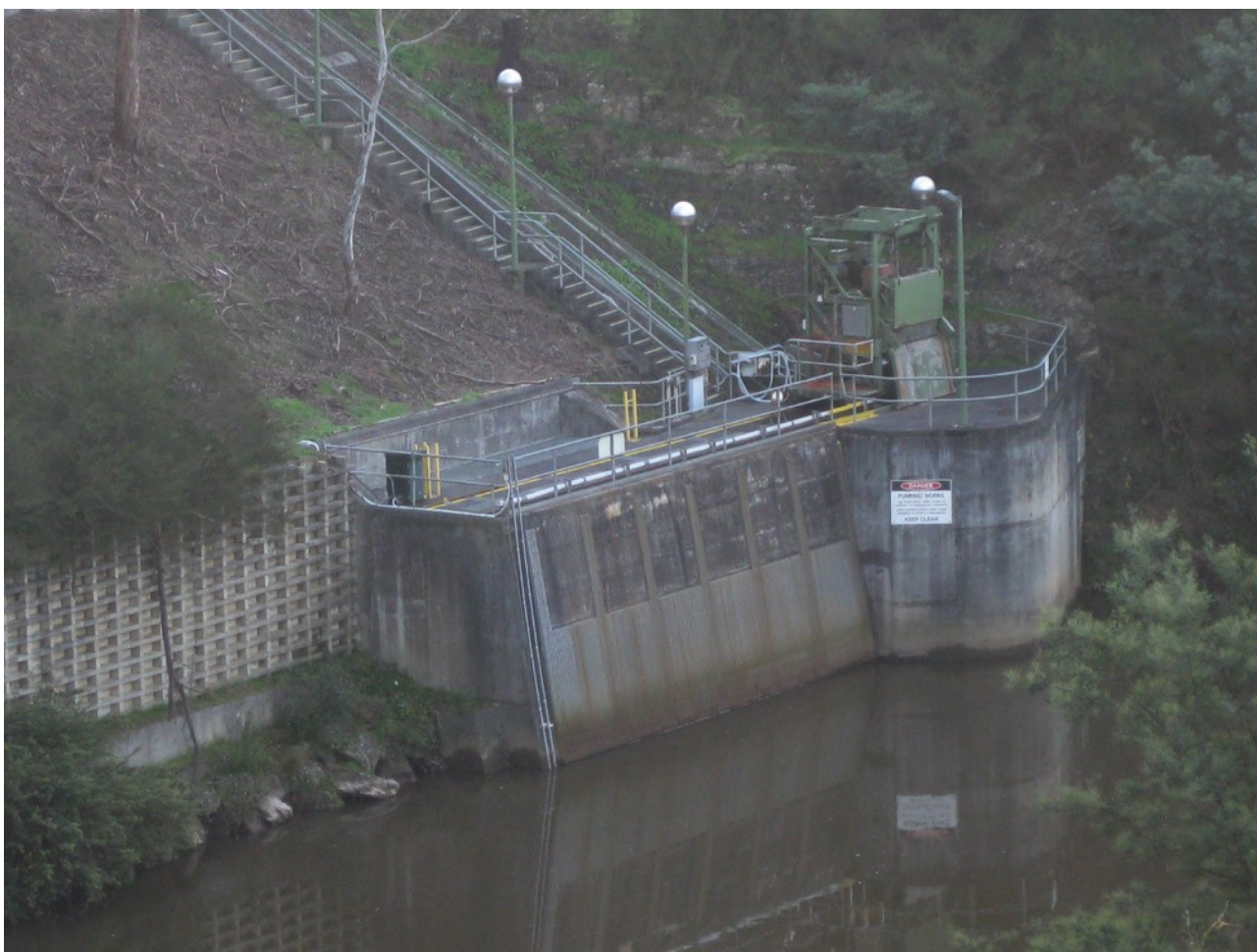
Photo June 2012: Water is pumped from the Yarra River at this location. Yering Pump House – Yering Gorge. 31 Positive Pesticide Detections were recorded by Melbourne Water at this location between July 23 2010 – August 11 2011 along with seven types of pharmaceuticals. Winneke Treatment Plant was never designed to filter out pesticides.
