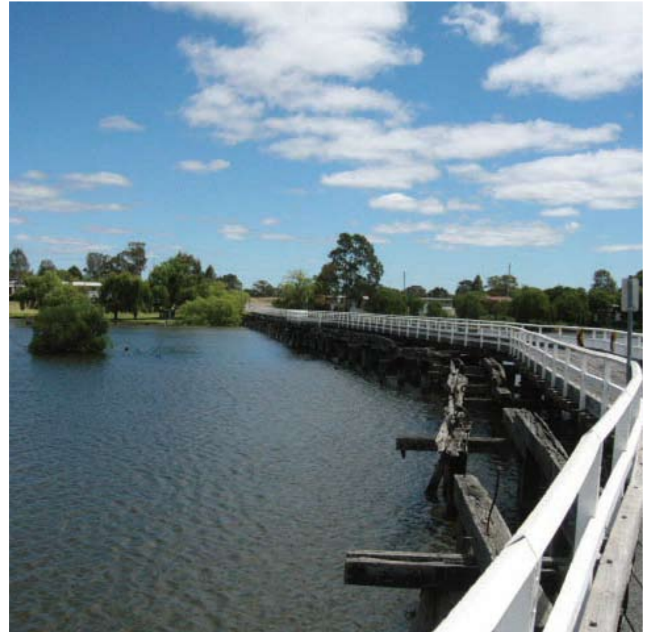
Kirwans Bridge at Goulburn Weir Backwater
